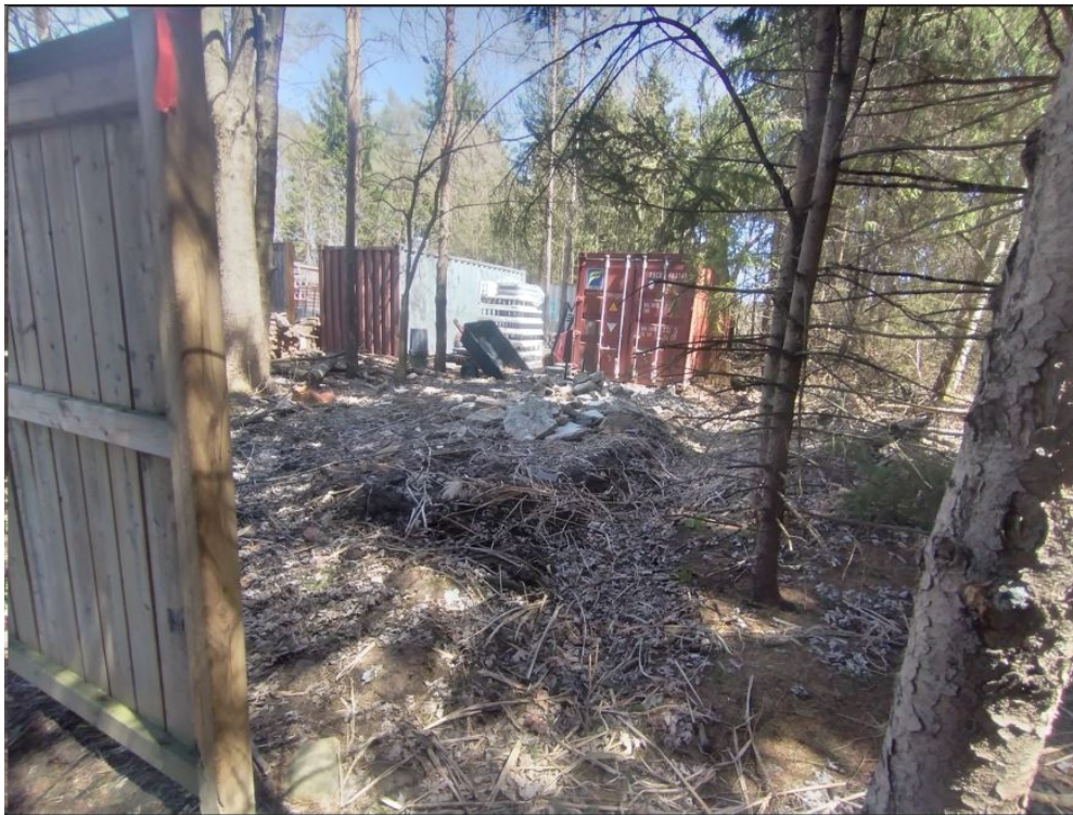
Fig. 9. Tree removal on adjacent property
