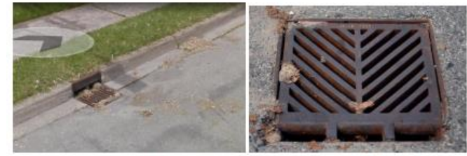
Figure 3-4: Existing Catch basin on David Street vs. Standard Catch Basin with OPSP 400.010 Grate (Source: Satellite Imagery @ 2022 Google)
